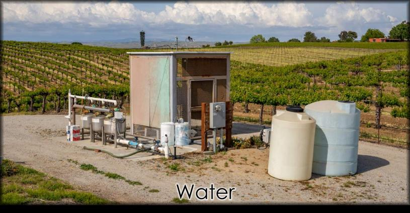
2 Wells: Irrigation: 950' Depth, 75 HP Pump (Est. 200 - 300 GPM) Domestic: 750' Depth, 3 HP Pump
